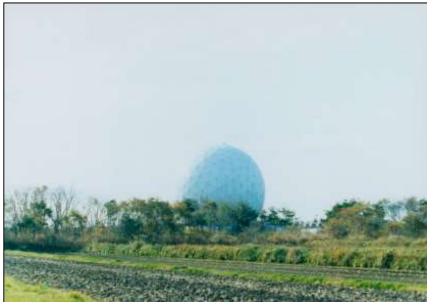
Plate 152 Radome with 18-metre Deep Space Tracking System (DSTS) antenna, Misawa, 1991
