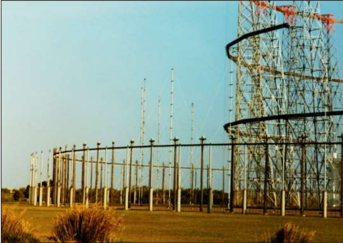
Plate 64 AN/FRD-10 CDAA at Camp Hanza, Okinawa, 27 April 1981 (Note outer ring of High-band antenna elements and inner ring of Low-band antenna elements)
