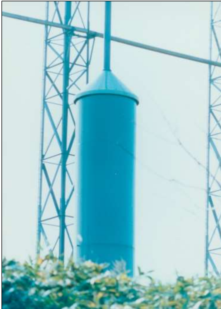
Plate 94 Low-band (2-6 MHz) sleeve monopole element, AN/FLR-9 CDAA, Misawa, 1991
