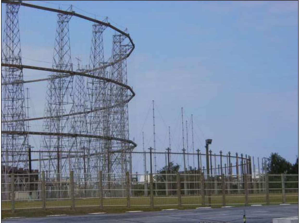
Plate 65 AN/FRD-10 CDAA at Camp Hanza, Okinawa, February 2003 (Note outer ring of High-band antenna elements and inner ring of Low-band antenna elements)
