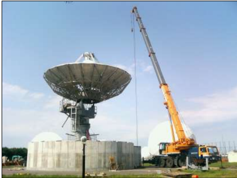
Plate 144 Installation of new dish/radome, Misawa, June 2007
