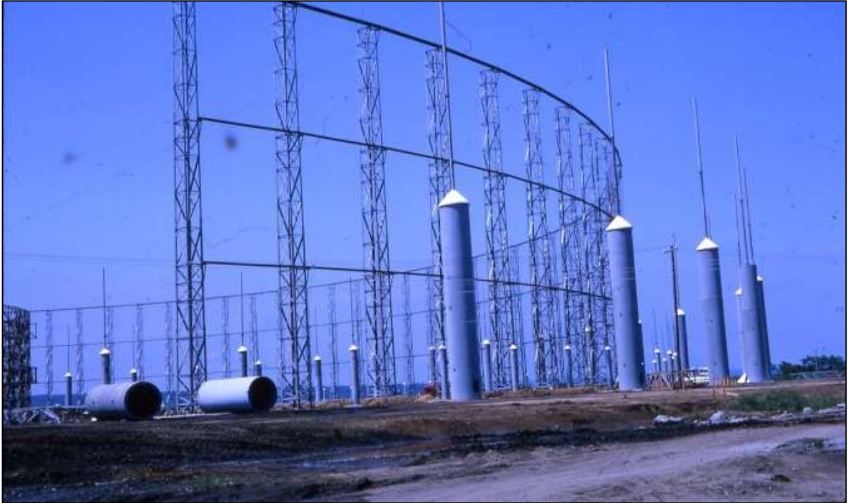
Plate 89 AN/FLR-9 CDAA under construction, Misawa, 1964
