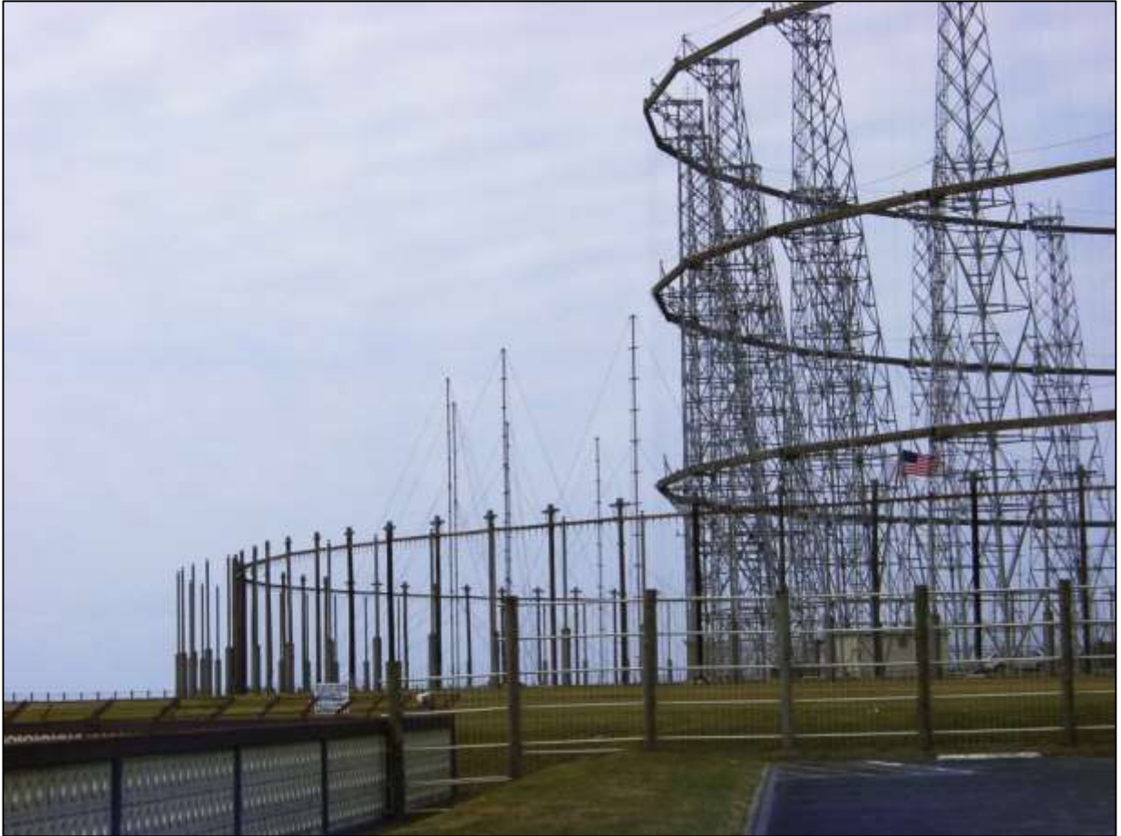
Plate 66 AN/FRD-10 CDAA at Camp Hanza, Okinawa, February 2003 (Note outer ring of High-band antenna elements and inner ring of Low-band antenna elements)
