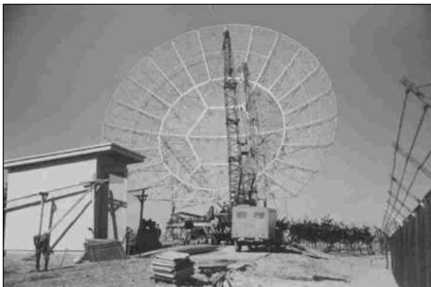
Plate 46 Dismantlement of ELINT dish at Sakata, 1962
